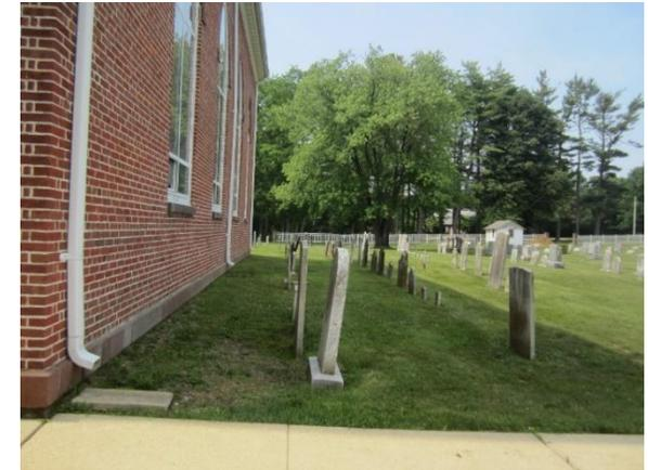
Roof runoff currently flows into six disconnected downspouts. Each downspout can be rerouted into planter boxes to reuse this runoff. A preliminary soil assessment suggests that the soils have suitable drainage characteristics for green infrastructure.
