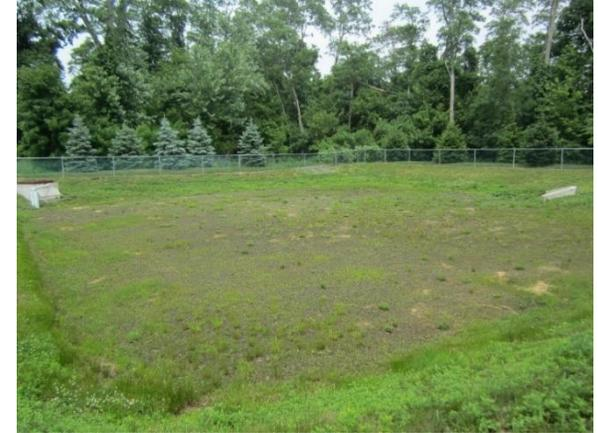
The building has directly connected downspouts. Most runoff is directed into a detention basin to the north. Pervious pavement can be utilized in the parking lot to capture and infiltrate this runoff. A rain garden can be constructed near the roadway to capture, treat, and infiltrate additional stormwater from the driveway. A preliminary soil assessment suggests that the soils have suitable drainage characteristics for green infrastructure.
