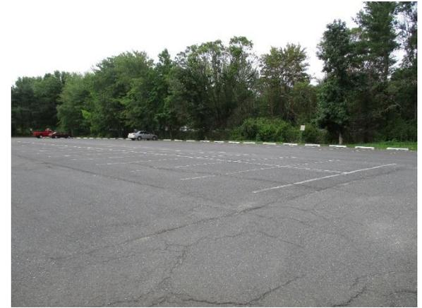
Most of the building has internal drainage. The front driveway drains into the roadway, and the parking lot drains into a swale near the highway. A rain garden can be installed in front of the building to treat stormwater from the driveway. Pervious pavement can replace parking spaces along the southwest edge of the parking lot to capture and infiltrate runoff. A preliminary soil assessment suggests that the soils have suitable drainage characteristics for green infrastructure.
