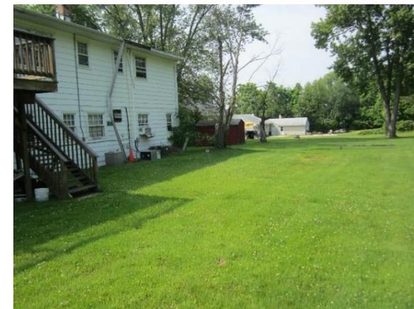
Roof runoff flows through disconnected downspouts into the parking lot, and to the rear of building. Parking spaces can be replaced with pervious pavement to capture parking lot and roof runoff. A rain garden can be installed in the rear of the building to capture, treat, and infiltrate roof runoff as well. A preliminary soil assessment suggests that more soil testing would be required before determining the soil's suitability for green infrastructure.
